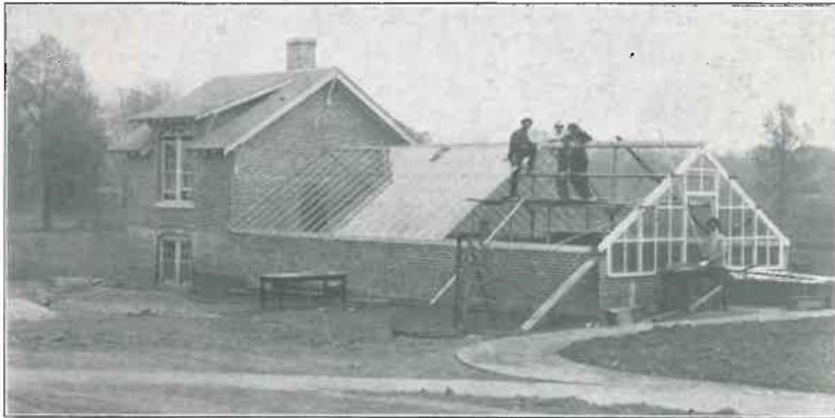
BOYS CONSTRUCTING GREEN HOUSE
